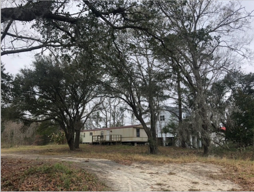
1- Existing mobile home on TMS-097
