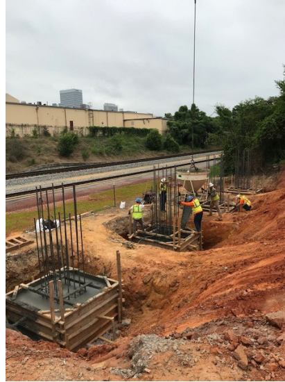
Innovista – Greene St. Ph. 2 Bridge Installation
