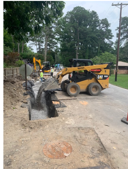
Harrison Rd. Sidewalk Drainage Installation
