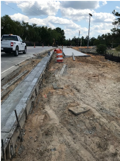
Polo Rd. Sidewalk Installation
