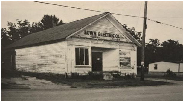
R.W. Frick Store Built 1908 and moved to its present location about 1950.
