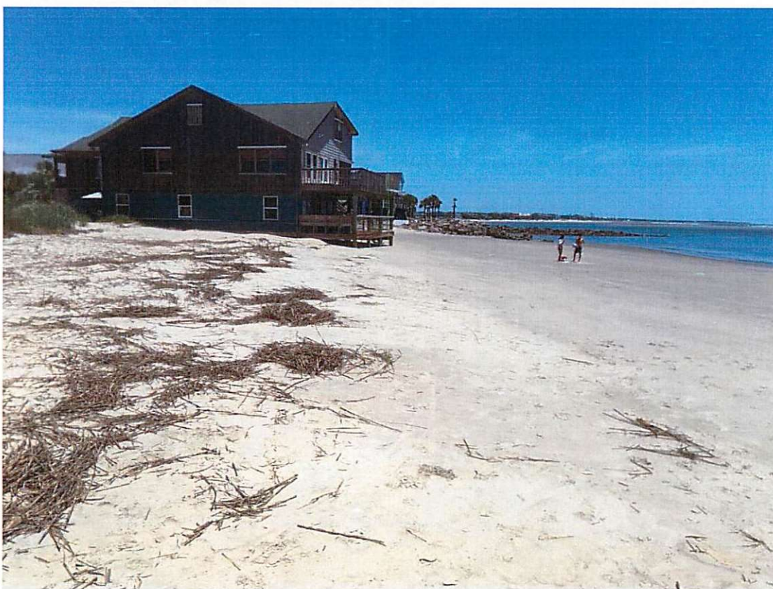
Figure 29. Ground photo taken at Monument 3085 looking northwest on June 6, 2019 (top) and June 2, 2020 (bottom). Notice the profile deflation under the deck in 2019 and backbeach recovery in 2020.
