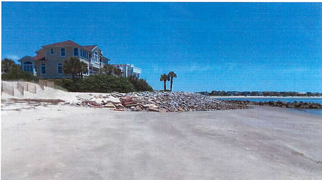
Figure 35. Ground photo taken at Monument 3092 looking north on June 6, 2019 (top) and June 2, 2020 (bottom).
