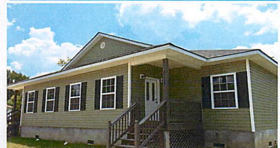
Pictured: New Construction for rental by the Town of Hollywood
