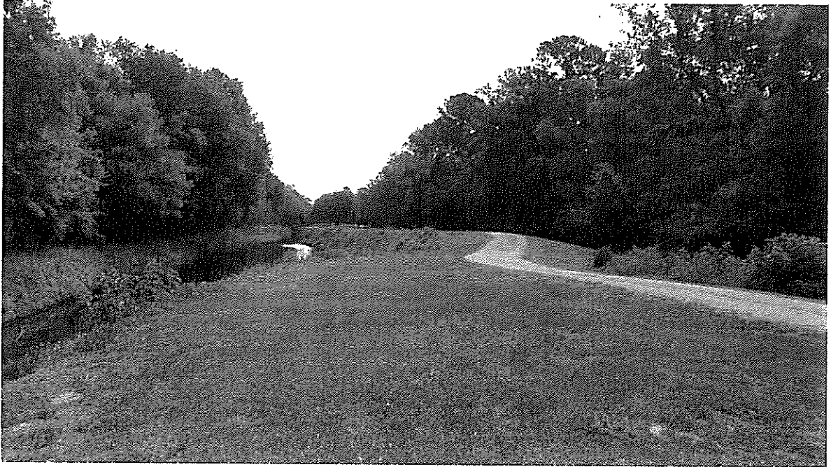
Mulberry Pond area (view East). Drainage canal varies in width and has multiple flow controls included along channel. New path will generally follow existing alignment due to limited room for adjustment.
