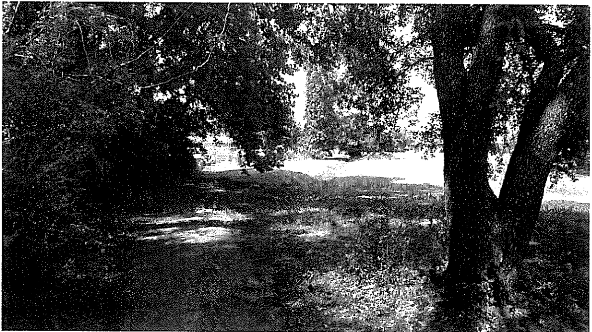
WAB, viewed towards Wappoo Road. Photo near rear of Limehouse Station property. Note root damage to narrow path.
