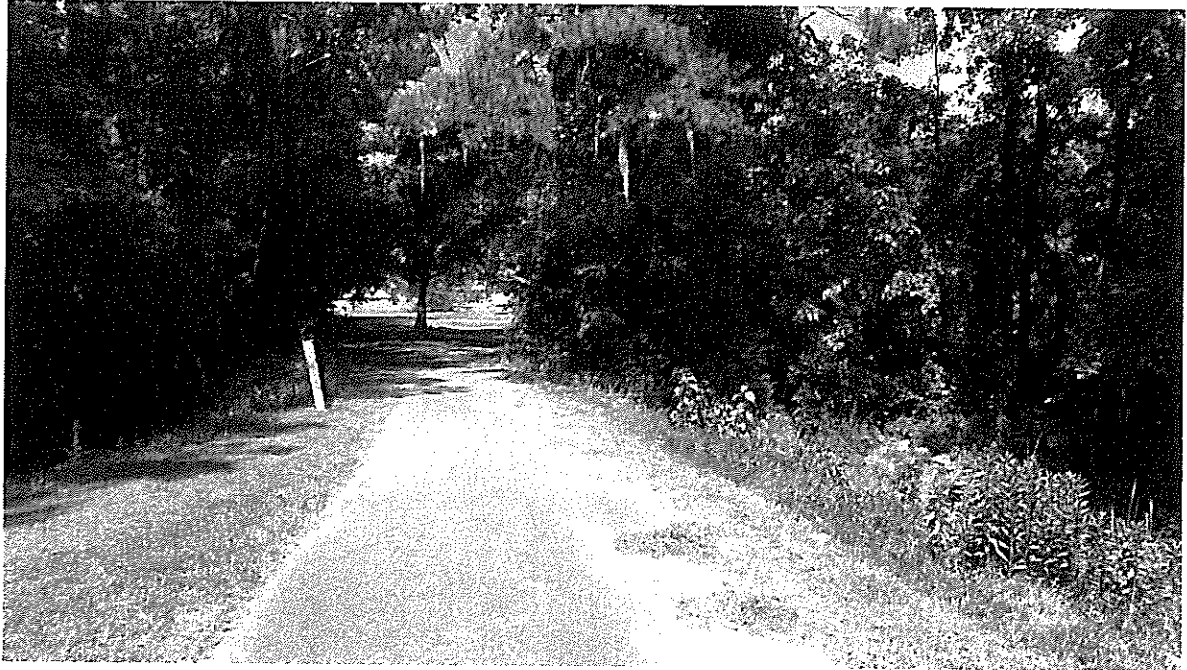
WAB at transition from Ardmore Drainage project (1995) to original path (1983). View west, with Limehouse Station property in center background. Path narrows from 8' shown to 6' original path near tree in center. Squares of grass from old post locations for low barrier.
