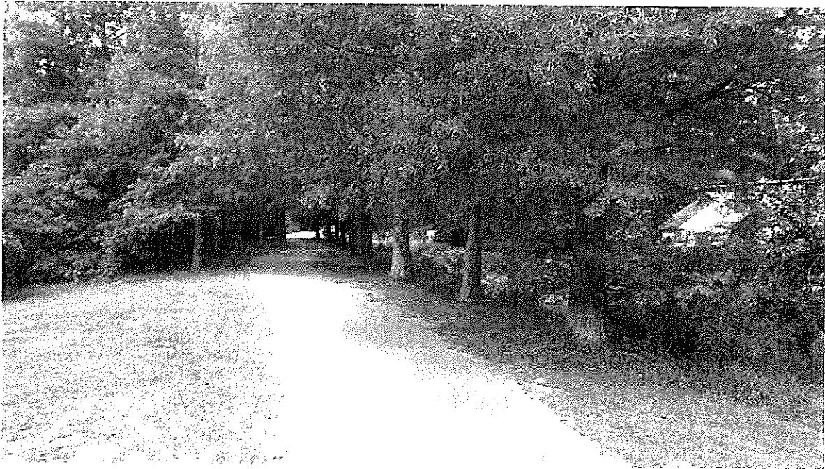
Bald Cypress grove (view West). Surprisingly little root damage in this shady stretch. Safety Barrier will be required on the right if the trees on the left are to remain.
