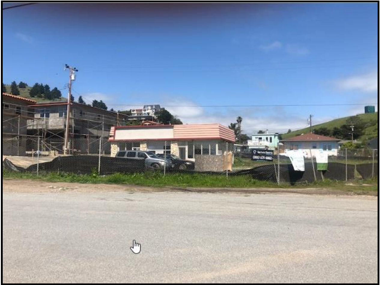
This view (dated approximately April 13, 2020) shows the (now-demolished) building on the property, looking East from Ocean Boulevard
