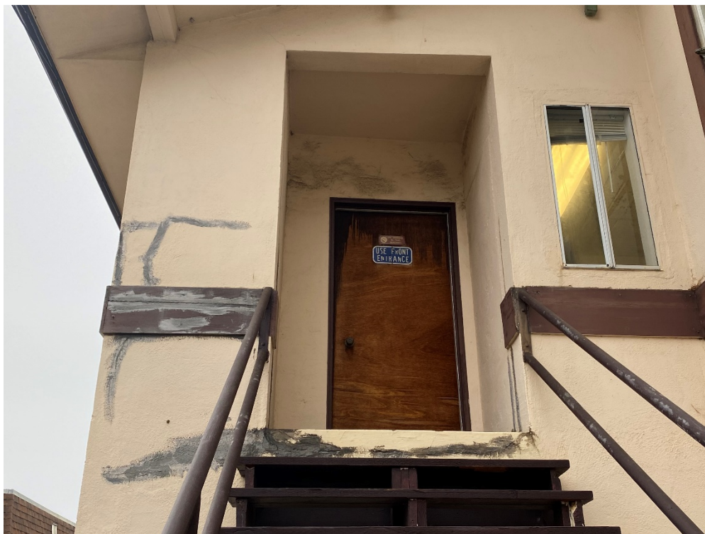
Distress Cracks on the outside of the building.
