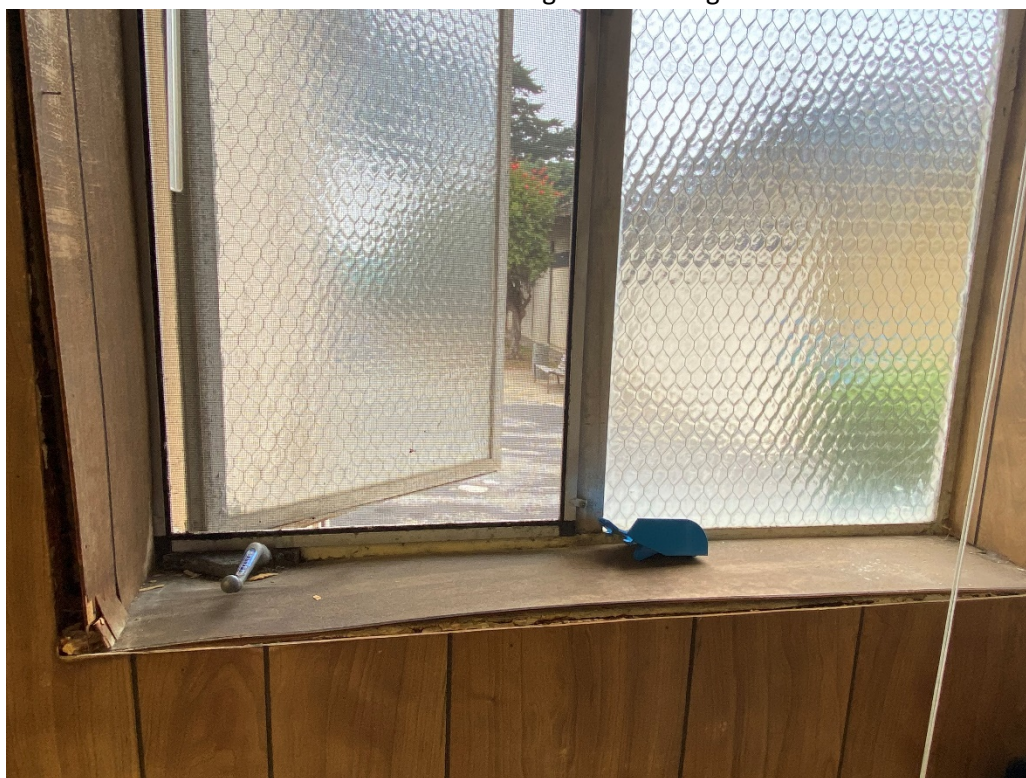
Window sills showing water damage.
