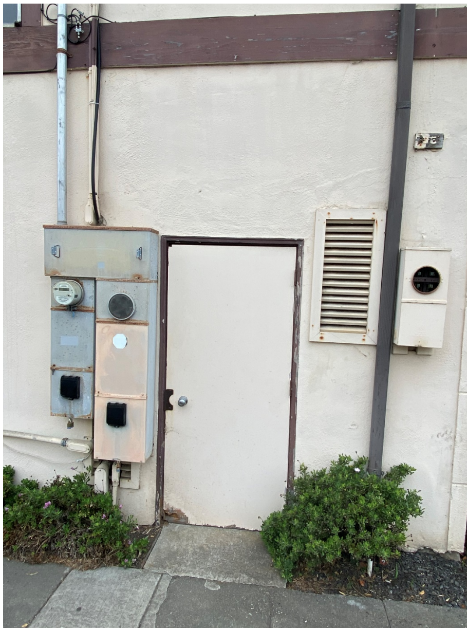
City Hall electrical boxes with abandoned electrical panels.
