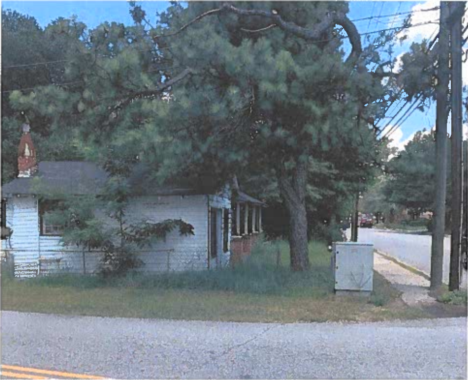
View of property from Pine St.
