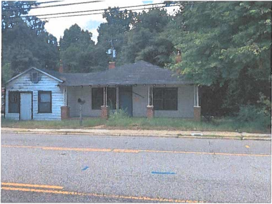
View of property from N. Main St.
