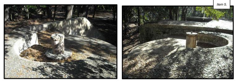
The parapet of Battery Fornance at gun #1. Left is looking north toward Battery Jesup, the right is looking south toward the #2 gun position at Battery Fornance. The large concrete column in the center is the pedestal on which the 4.72-inch gun was mounted.
