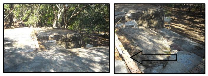
Battery Fornance #2 gun position. (Left) This is looking north toward the traverse and gun #1 position. (Right) This is a detail of the #2 gun position. The arrow is pointing to a low course of bricks that surrounded the gun position. The concrete pedestal was removed. The few bricks are the only remnants of the house that was constructed on top of the #2 gun position.
