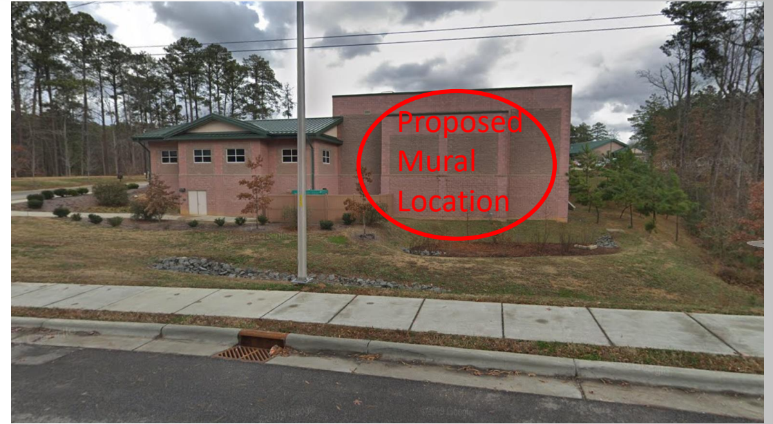
Apex Public Works Building – Route 55
