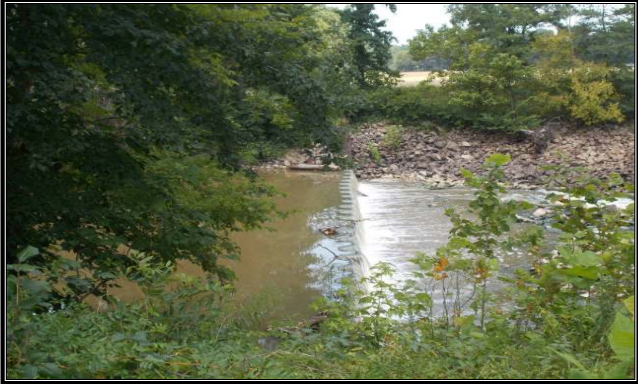
RIPARIAN BUFFER / WEIR REPAIR AREA
