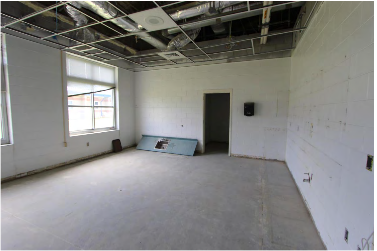
Room A108, casework, plumbing fixture, and grid demo'ed
