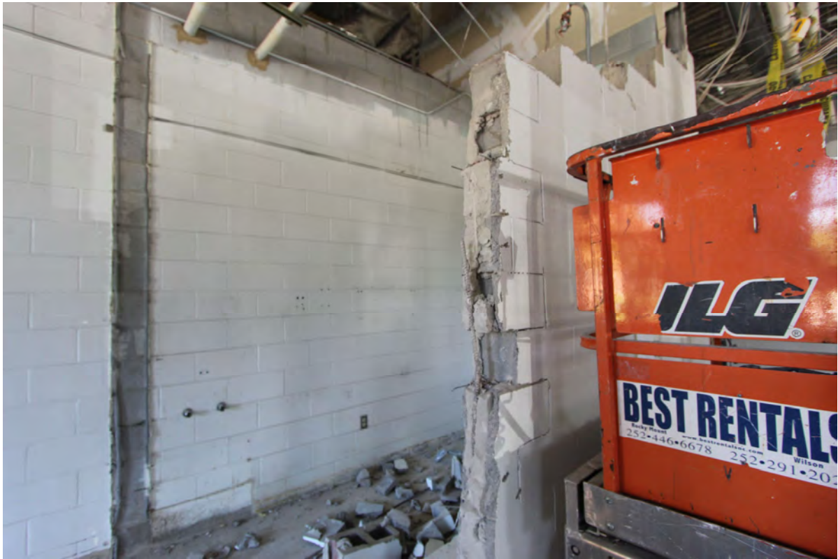
Block walls grouted solid and reinforced with rebar
