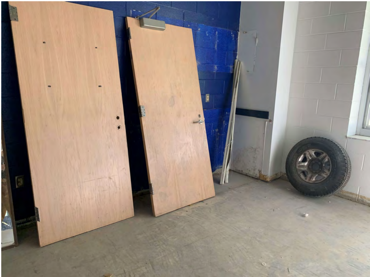
Casework in Room A104, was removed and needs to be put back or replaced
