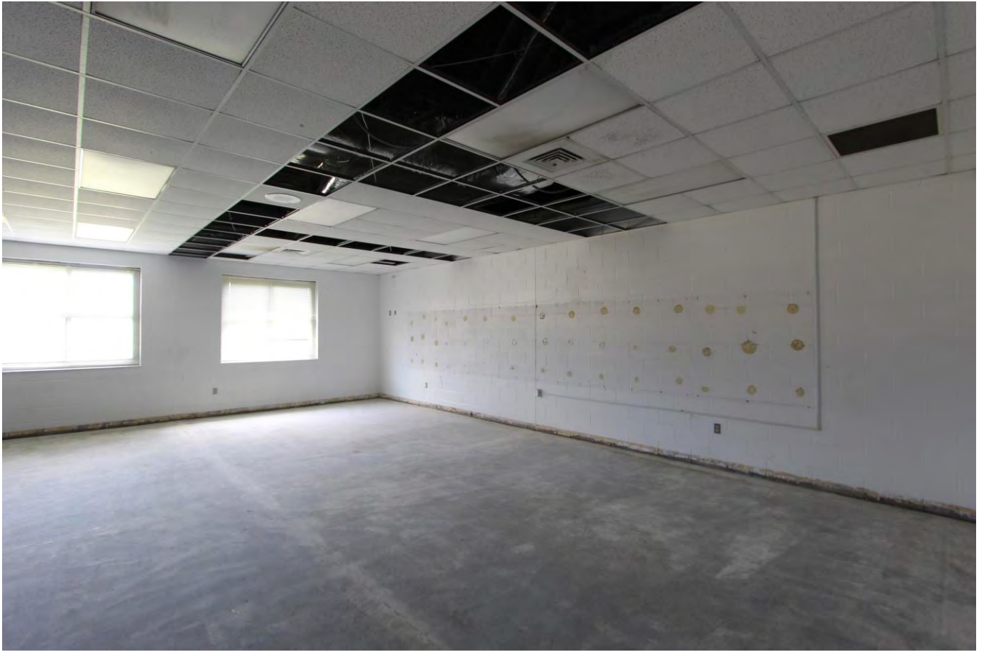
Ceiling tiles being removed to prep for new stud walls
