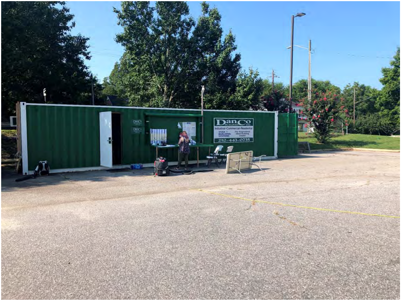
Job Trailer on site. Awaiting temp power and data services.
