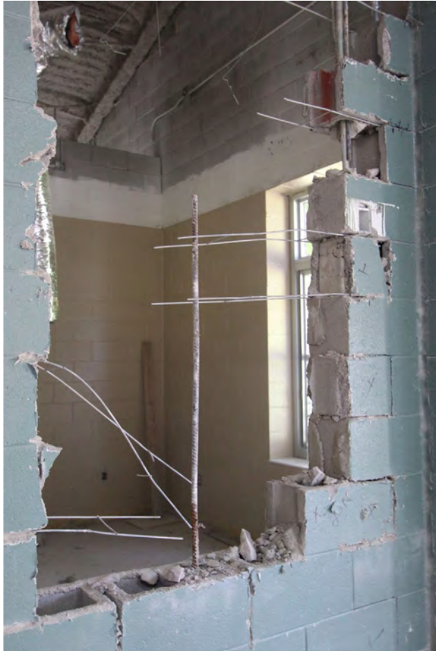
Block walls grouted solid and reinforced with rebar
