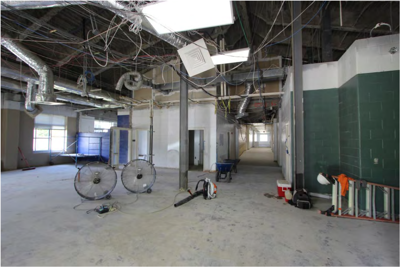
Demolition of Block wall progress near front entrance
