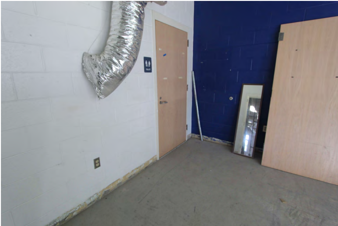
Door to Bathroom A104A, has been replaced.
