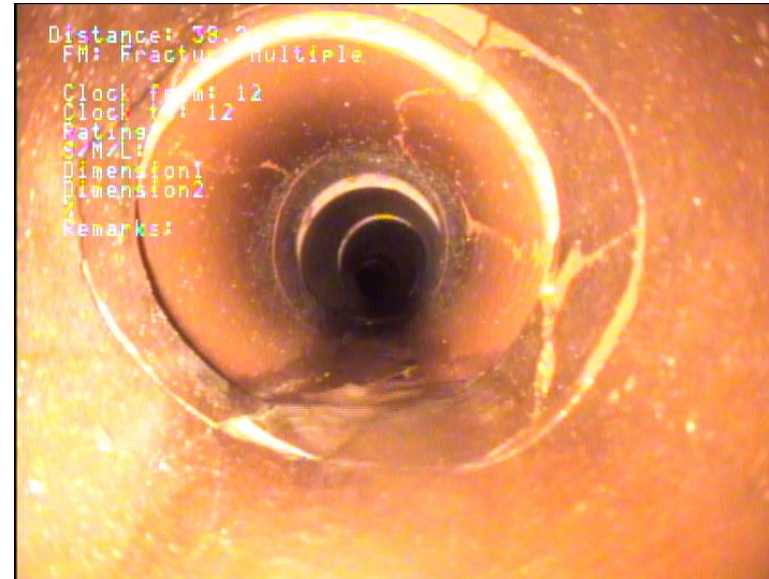
Severe Offset/Fracture
