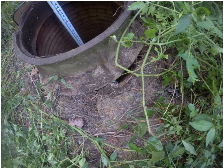
Hole in Frame (allows inflow)
