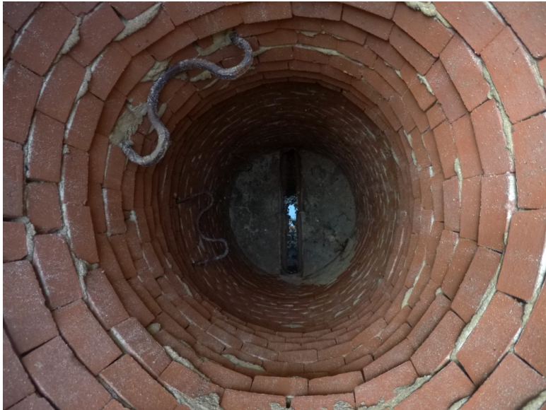
Typical Brick Manhole
