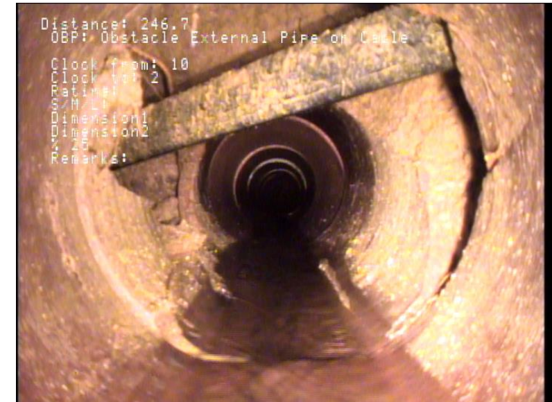
Cable installed through Sewer Pipe
