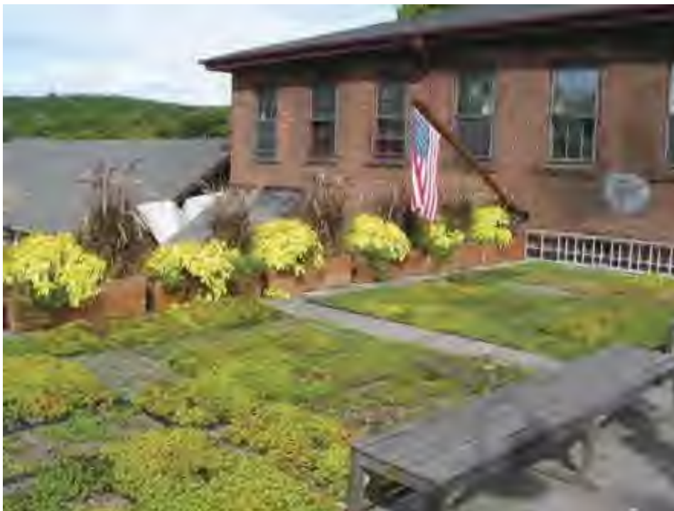
Figure 4.20. Green roof (photo: Center for Watershed Protection, Inc.)
