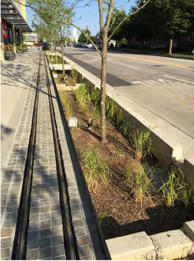
Figure 4.5. Example streetscape bioretention.
