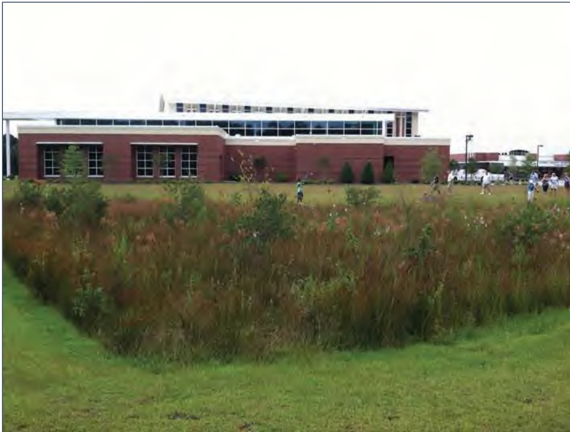
Figure 4.50 Stormwater Wetland at Carolina Forest Recreation Center, Myrtle Beach (photo: Kathryn Ellis).
