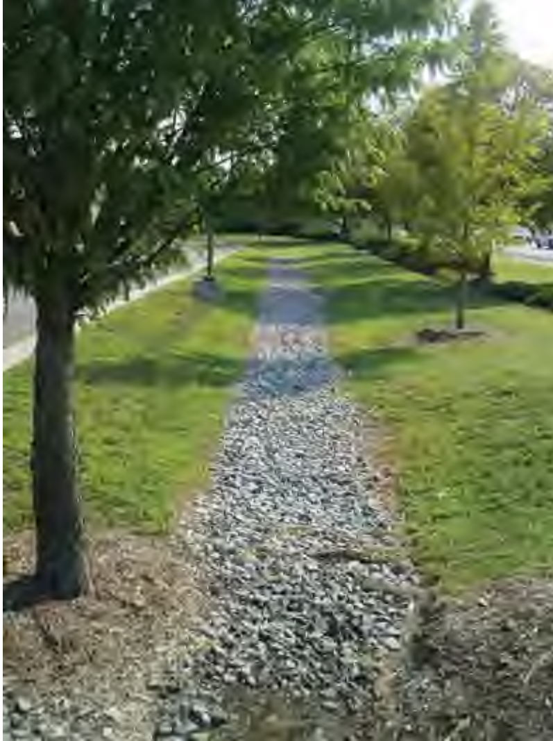
Figure 4.16. Infiltration practice in median strip.
